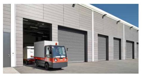
The **convenient operation via operator** is the best solution for doors with a high opening frequency.
